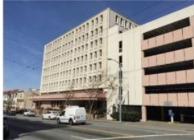
The fully leased medical office building is located in Presidio Heights.
