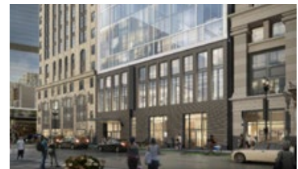
180 W Randolph Hotel mixed-use redevelopment ±0.17 AC CHICAGO, IL
